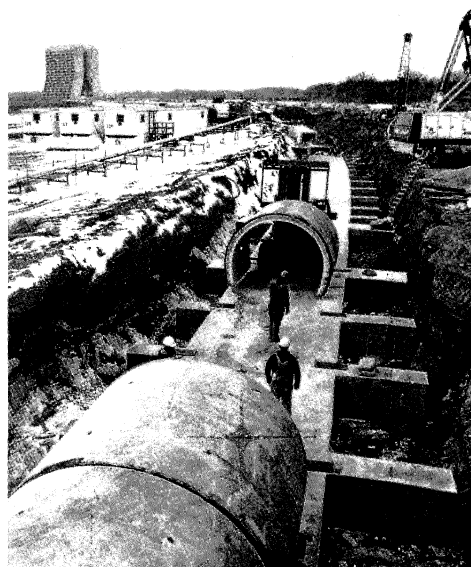
3 — old tunnel sections make up the second floor
