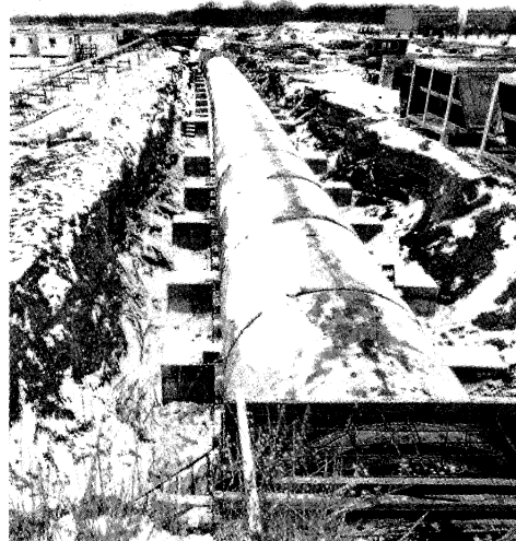
4 — second floor takes shape
